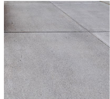
Plate 4-15 Example of concrete pavers/hardstanding
